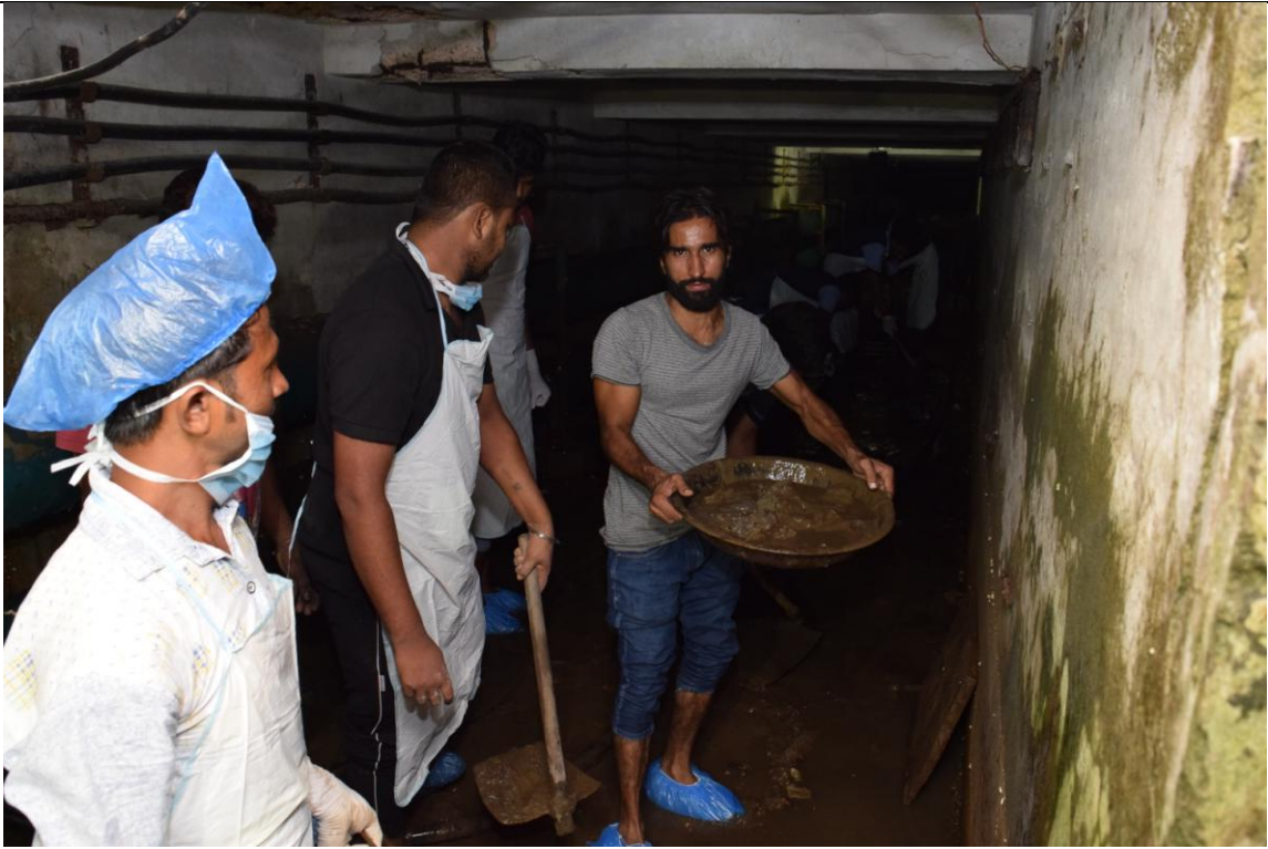
Cleaning drive of basement (Main OT), SJH
