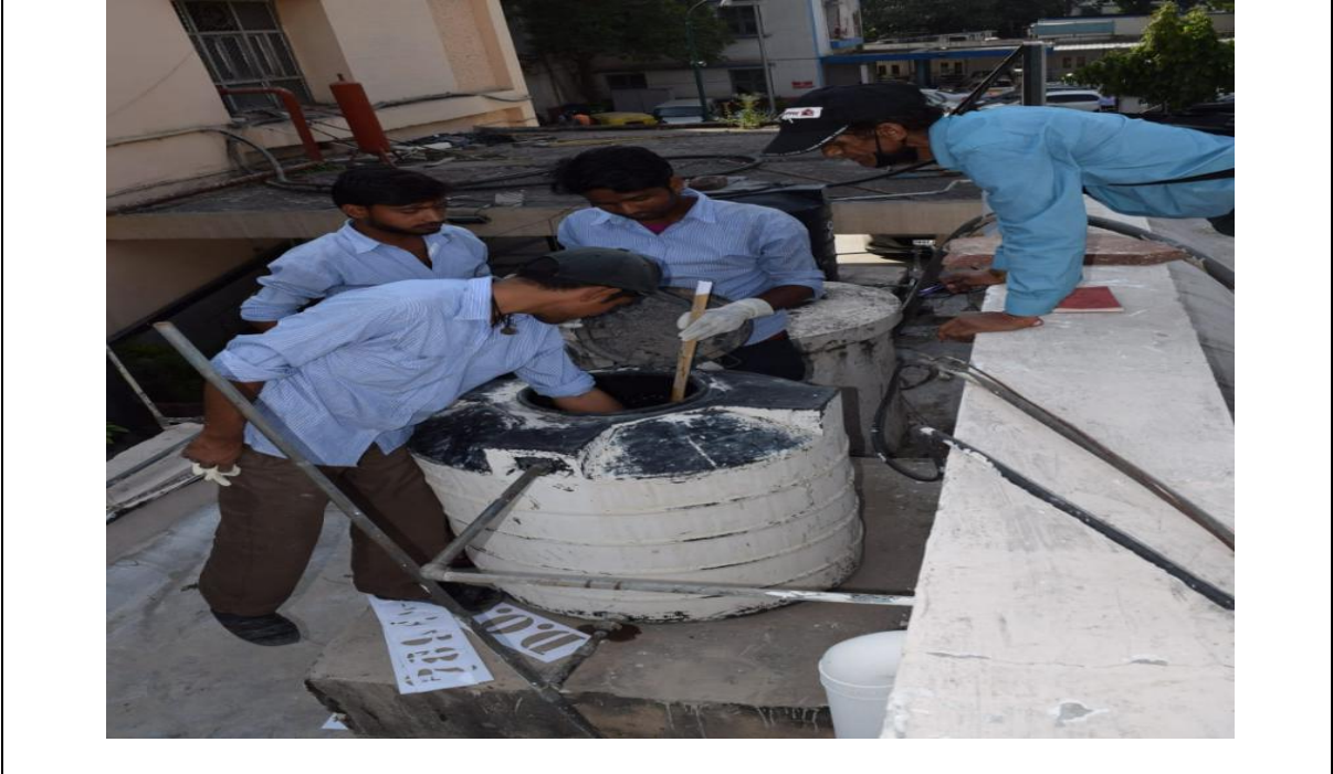
Cleaning of overhead tank, SJH- 19/09/2018
