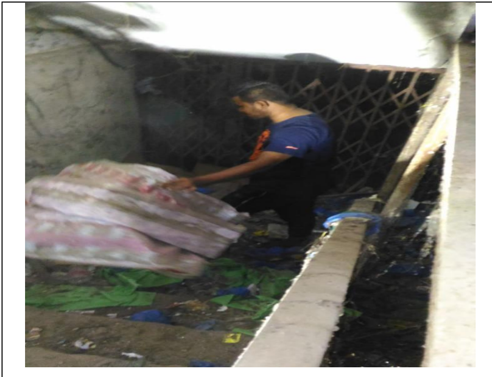
Cleaning drive of basement CSSD, SJH- 20/09/2018
